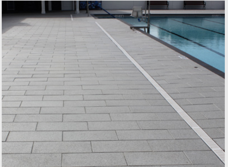
Eisenhower Recreation Center | The Villages, FL | Frontier Pavers
